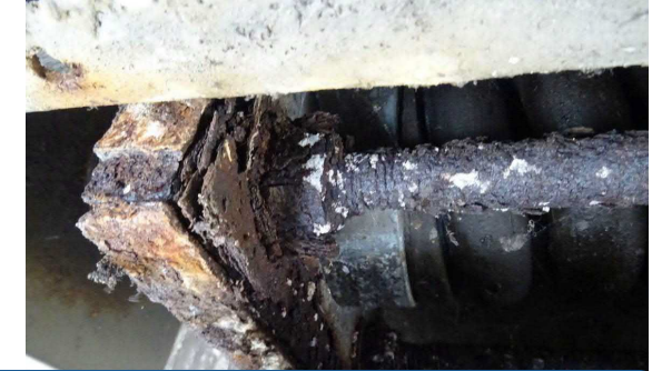
Gallows Corner Flyover (steel fatigue) Daily users – 38,000
