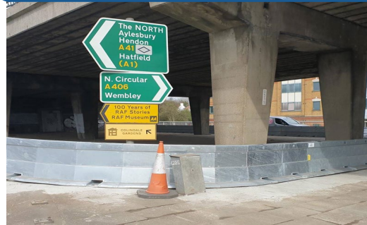
Brent Cross Structures (all over structural condition – very poor, temporary parapets in place) Daily users – 175,000
